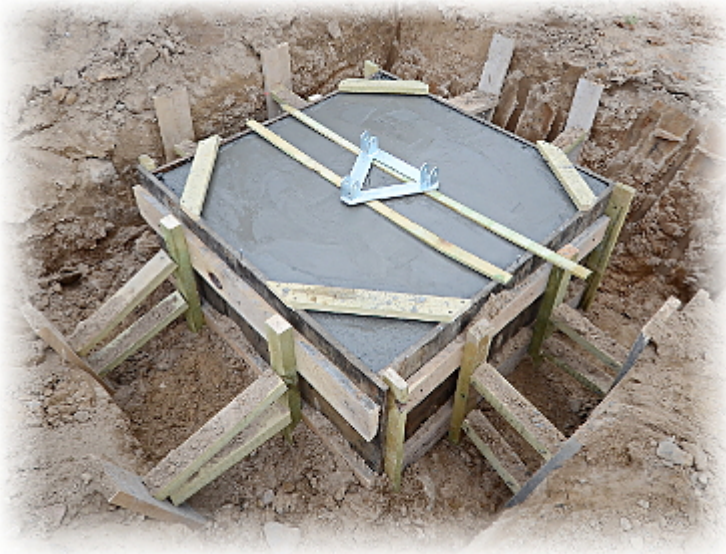
Ready foundation with the set mast:
