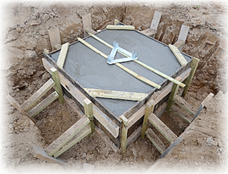
Ready foundation with the set mast:
