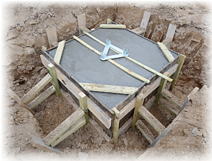
Ready foundation with the set mast:
