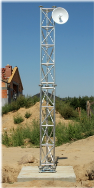
Prepared form-work for the foundation of the mast:
