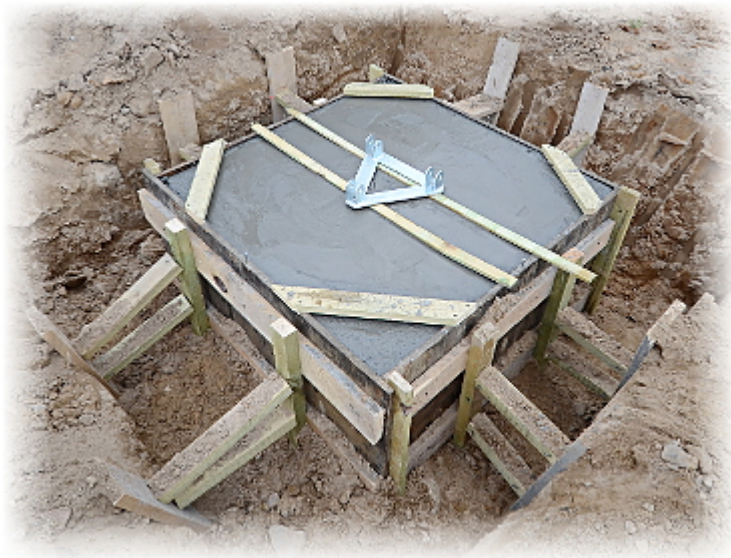
Ready foundation with the set mast:
