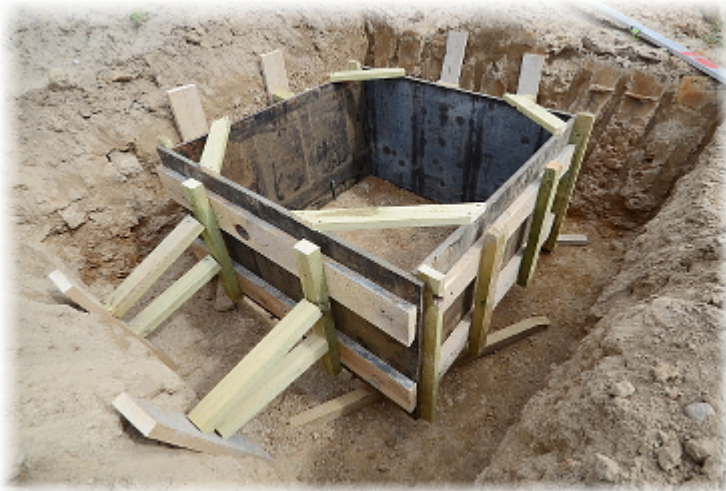
Poured foundation of the mast with embedded anchor and established base
