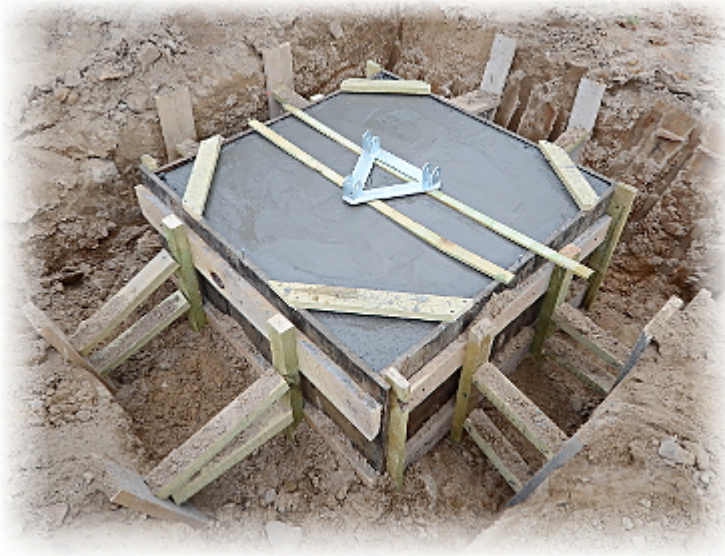
Ready foundation with the set mast:
