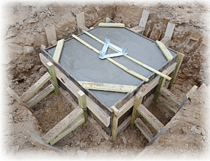
Ready foundation with the set mast
