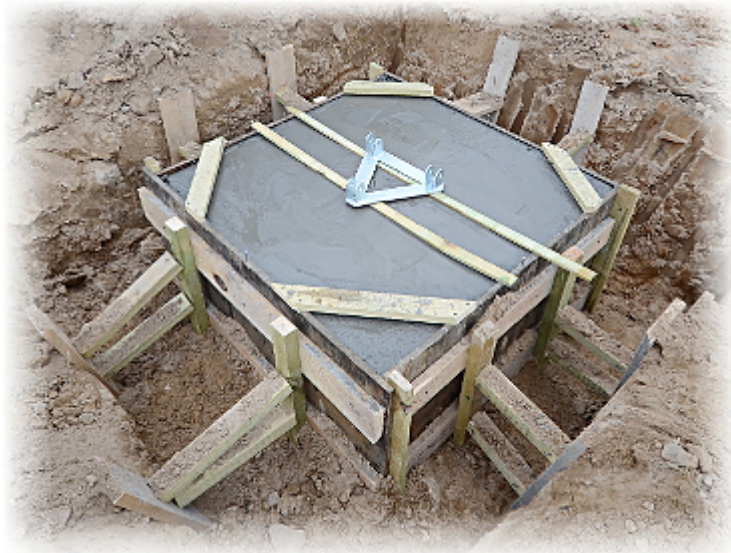
Ready foundation with the set mast:
