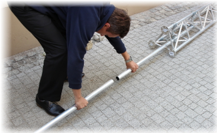
Pipe masts are combined on a wedge:
